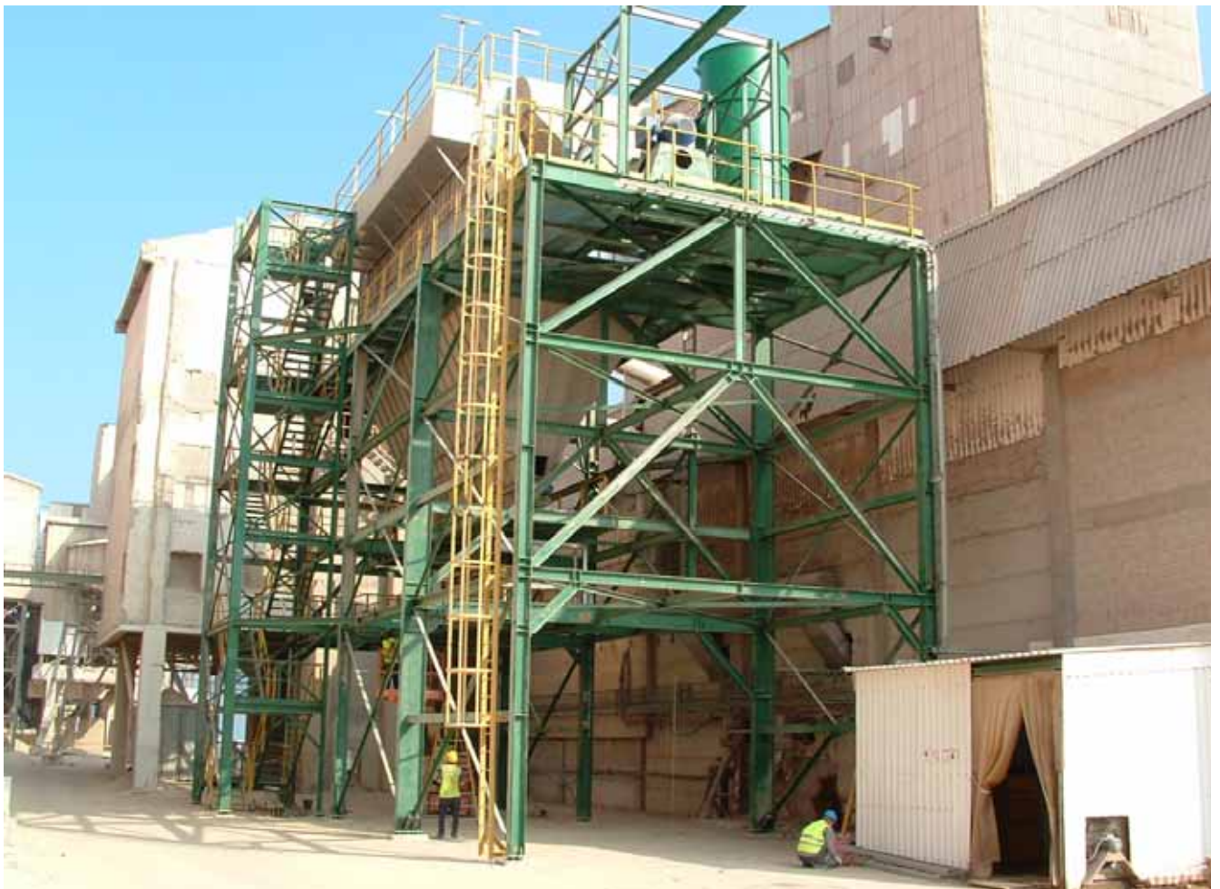
Potash Unloading pit Ashdod port 110,000 m 3 /h - Under Construction September 2008
